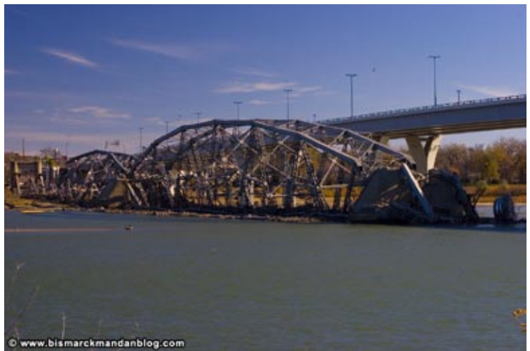
The remainder of Bismarck-Mandan's historic Liberty Memorial Bridge has come down.
